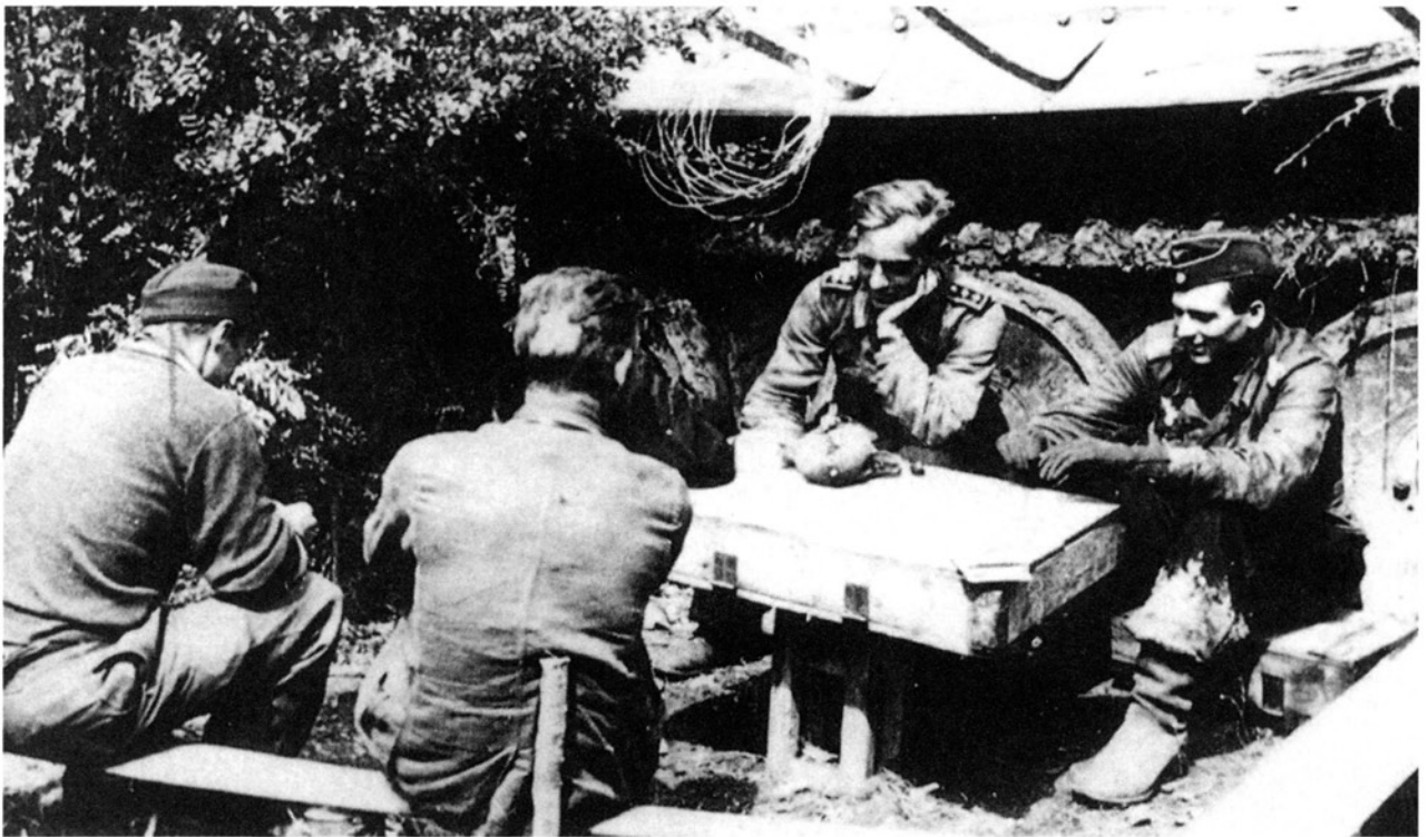
Leutnant Cūsow of the 2./schwere Panzer-Abteilung 503 enjoys a conversation with some of his men at the assembly area near Toloknoje. Some flat iron bars have been welded on the track mudguards for the attachment of barbed wire. This was done in an effort to discourage enemy tank-hunter/killer teams from attempting to climb on the tanks. RUBBEL
