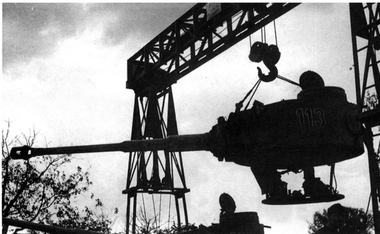
After the decision to stop the offensive at Kursk, the battalion had little time to get its broken-down or battle-damaged tanks operational again. The turret of Tiger 133 is lifted by the 15-ton portal crane on 30 July 1943.
