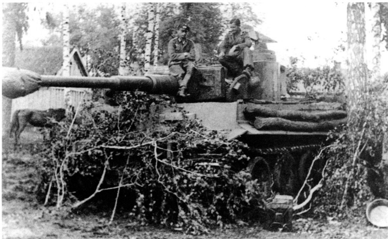
Many tanks of the battalion carried at least one wooden beam on the hull side. Sometimes a beam or beams were found on both sides of the tank. These were used to help a tank to sometimes free itself without outside assistance when bogged down. MÜNCH
