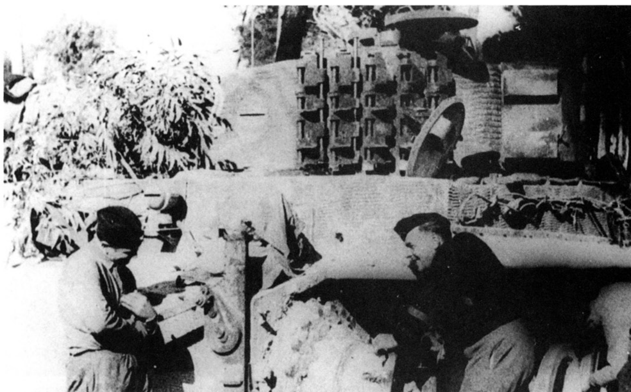
Since most of the tanks were immobilized by mines, major repairs needed to be effected to the running gear.
