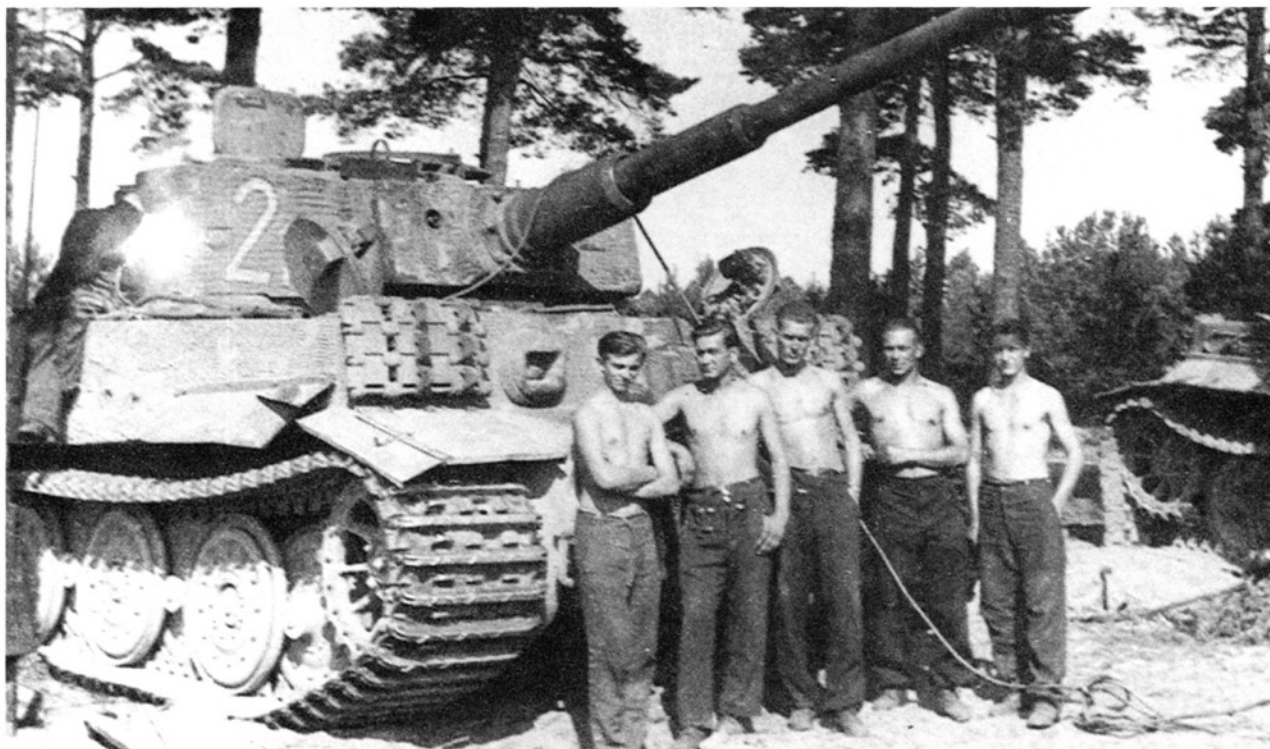
After arriving in the Olesko area, the 2./schwere Panzer-Abteilung 507 has attachments for mounting track links to the sides of the turrets added. HÜPFEL
