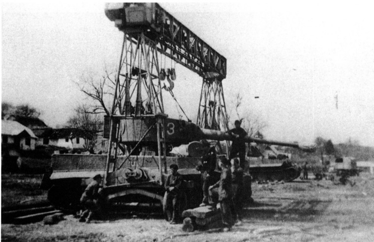
After the engagements around Olescha, the battalion's tanks were in urgent need of repair and maintenance. The tank of one of the platoon leaders of the 1./schwere Panzer-Abteilung 506 has its turret hoisted by the portal crane. VOGEL.
