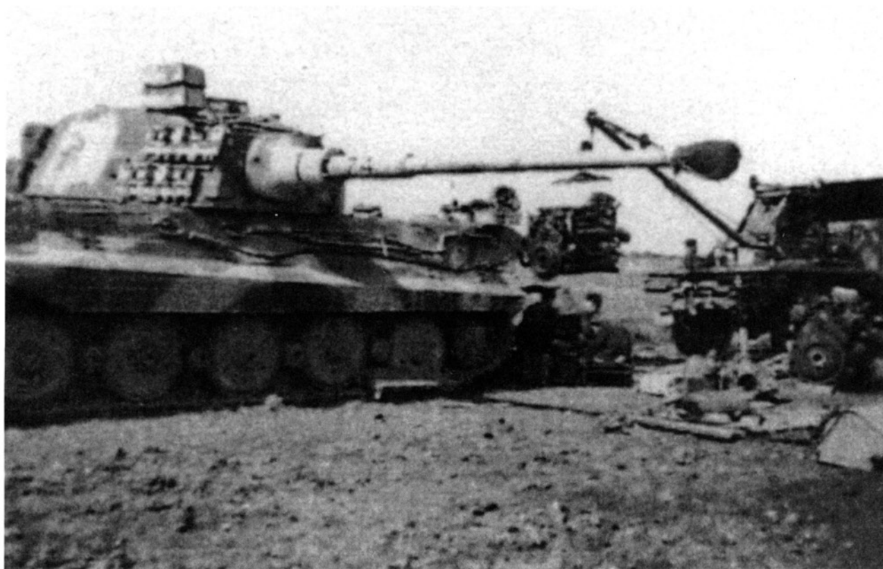
These three photographs show an engine being changed on a Tiger II. KRÖNKE
