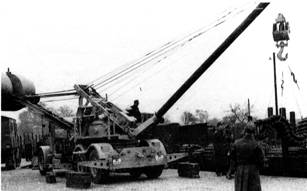
The combat tracks were delivered separately and unloaded by means of a crane. HARTMANN
