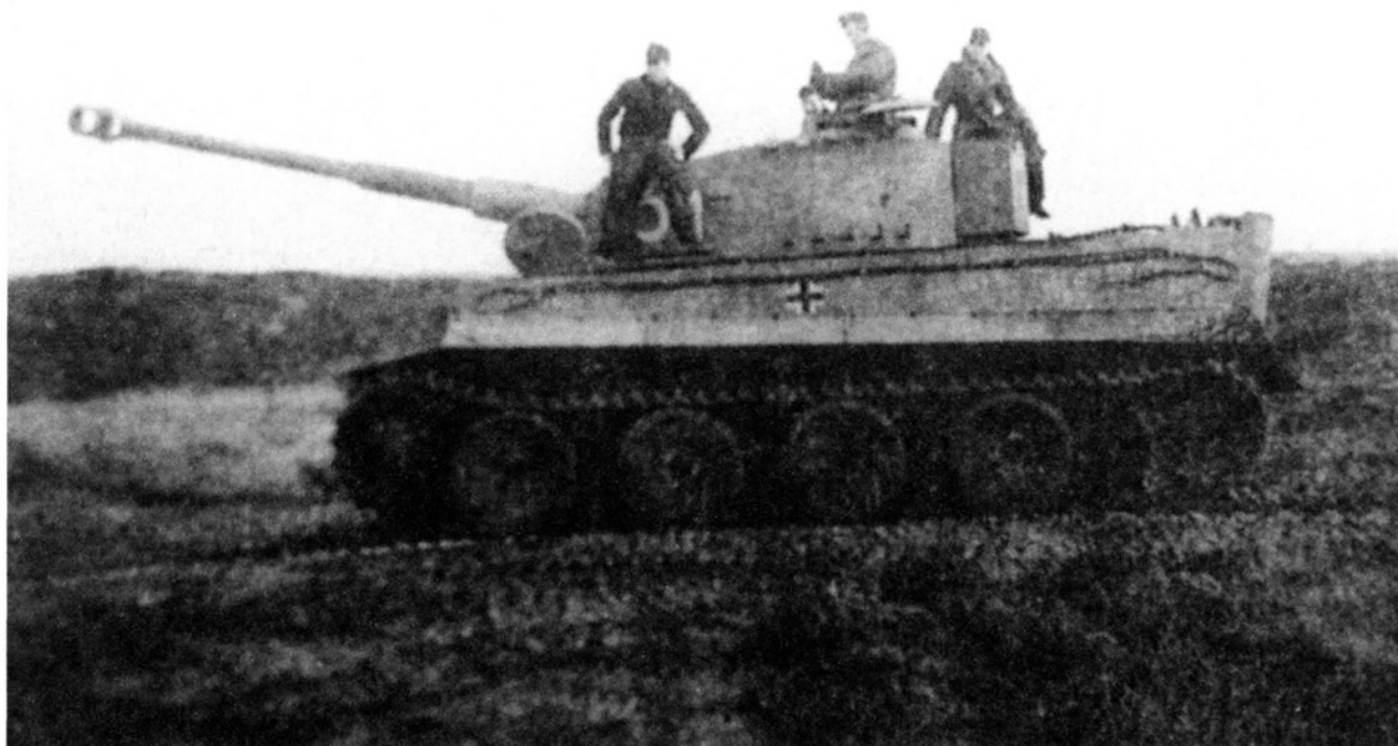
The battalion received several versions of the Tiger. On Tiger 311 we see a middle version with the later-style commander's cupola but with the earlier rubber-rimmed roadwheels. SCHNEIDER
