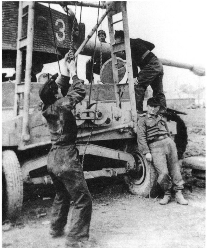
While the maintenance team lifts the turret, the tank commander observes in a relaxed fashion. VOGEL.
