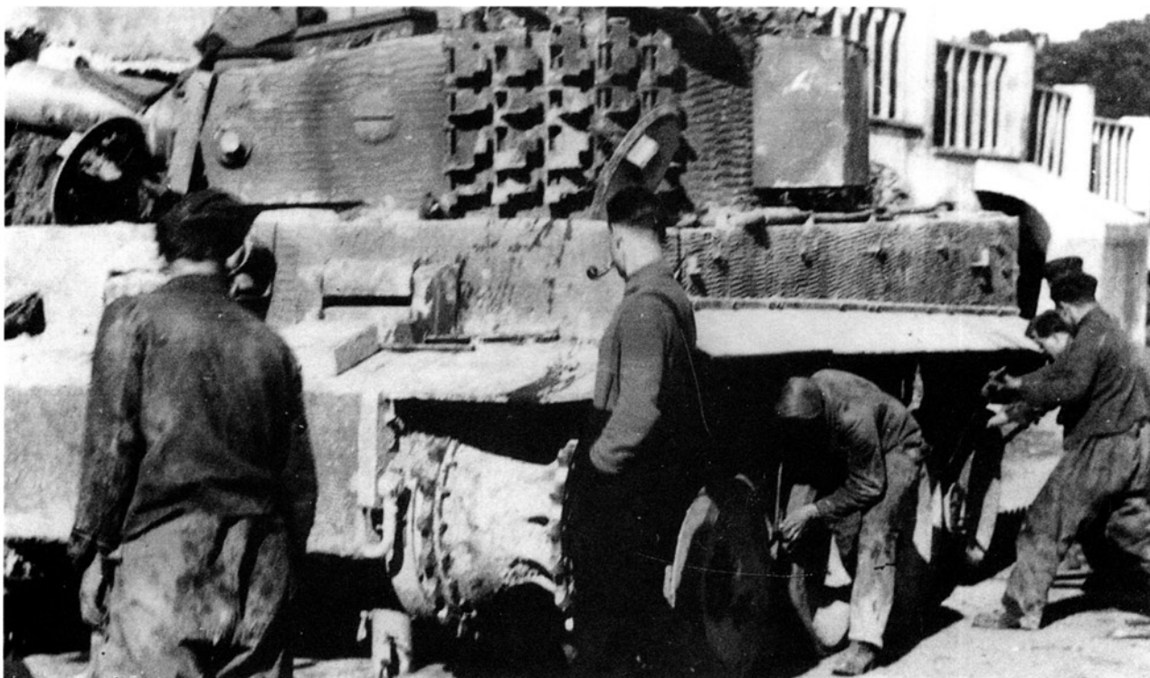
The damage suffered to the suspension on this Tiger was scheduled to be repaired at Forte Tiburtina. HIRLINGER
